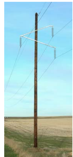
Typical 144 kV single-pole "wishbone" design
